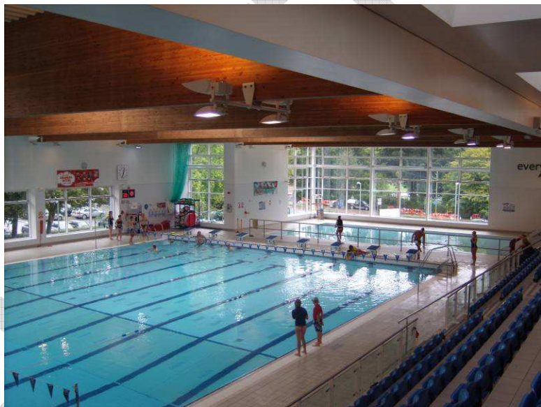
Woodside Leisure Centre: the 25 m x 8 lane pool. Most of the Borough's indoor facilities – public, school and commercial – are recently built and of high quality
